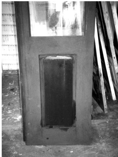
Figure 3 Maintenance of an old door, after nine years, with boiled linseed oil or linseed-oil wax.
